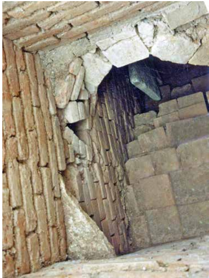
(a) Isometric view of the sarcophagus (2.38 m long \times 1.32 m wide \times 1.25 m deep) and its lid (13 cm thick) in Tomb III burial chamber; (b) stairs descending into the outer chamber of Tomb III. Note the remnant of a horizontal limestone sealing slab at lower left and the limestone door to the burial chamber in the open position at upper right. Note also triangular niche in west wall, center left
