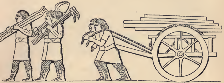
Cart with Ropes and Workmen carrying Saws, Picks and Shovels, for moving colossal Bull (Kouyunjik.)
