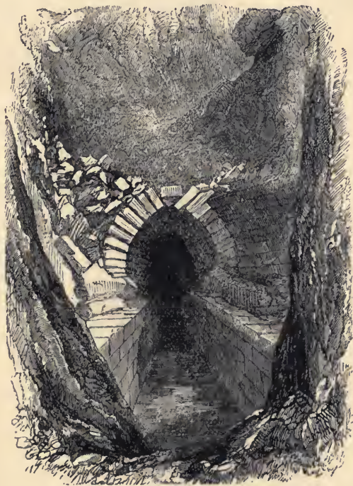
Vaulted Drain beneath South-east Palace. (Nimroud.)
