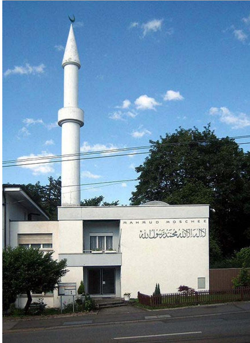
Mahmood Mosque, Zürich
